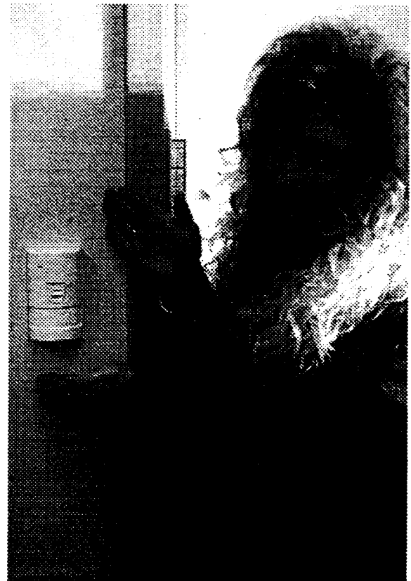
Occupancy sensors are often a good energy conservation measure.
