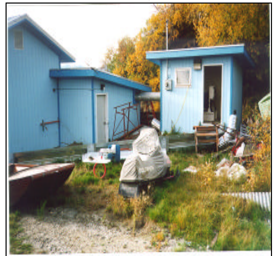
Wastewater treatment plant in Kiana, AK
