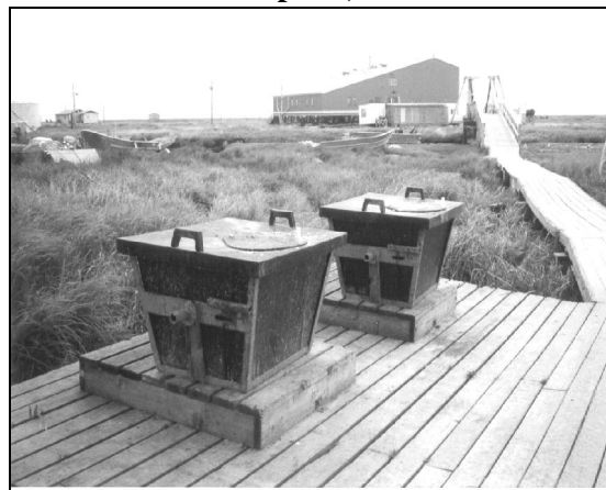
“Honey Bucket” haul station in Kipnuk, AK
